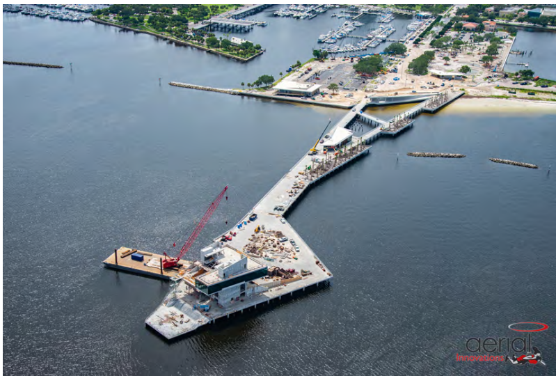
Figure 3.3. St. Pete Pier Construction in September 2019
